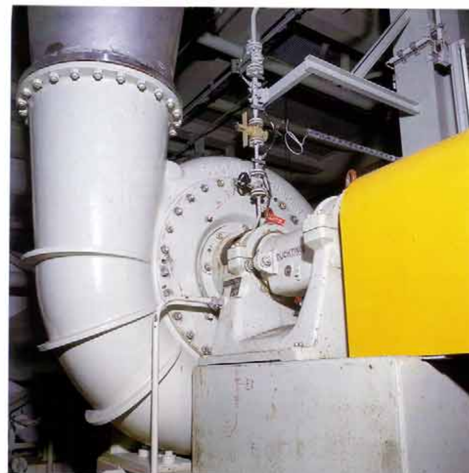
ROWA 800.106 An absorber-recirculating pump installed in a flue gas desulfurization plant
